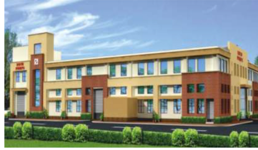
Roto Manufacturing Plant
